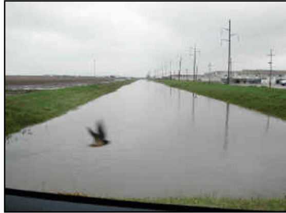
Wood River Diversion Project's main channel during 2005 flooding.
