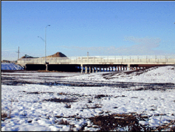
Locust Street Bridge. One of five that was built as part of the diversion project.
