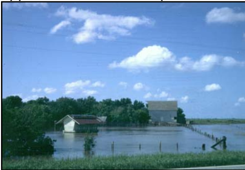
A flooded Hall County farm in 1967.
