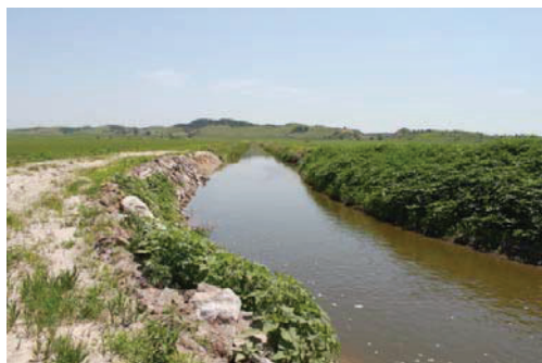
(Spring 2014): Completed section of canal holding water.
